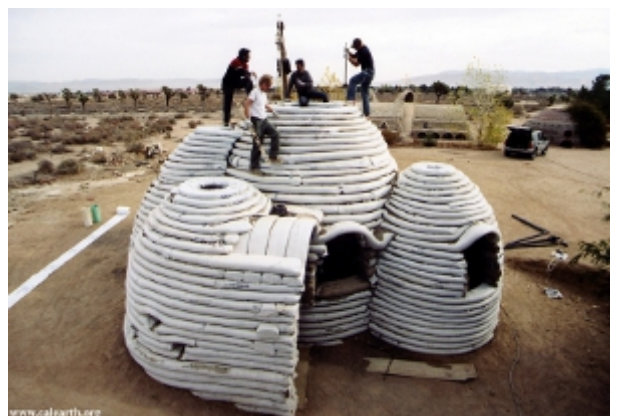
A typical SuperAdobe structure (Photo: Cal-Earth)
