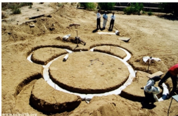
Foundations of a SuperAdobe structure (Photo: Cal-Earth)
